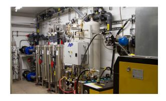
Ozone oxidation is one of the most effective water treatment processes and is environmentally friendly as ozone is produced onsite from oxygen and reverts back to oxygen after reacting with contaminants.
